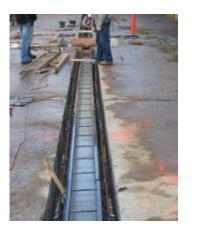
Aquaduct custom 8" trench drain with ductile iron grates
