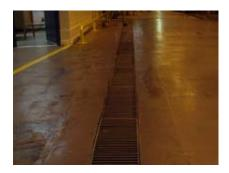
Lucerne Foods realized the need for trench drainage when they washed down the plant floors. To meet the hygiene requirements in food processing, the floors are regularly washed down with sodium hydroxide and need a trench system that was able to withstand this chemical exposure. Aquaduct custom trench was more than capable of meeting their needs.
